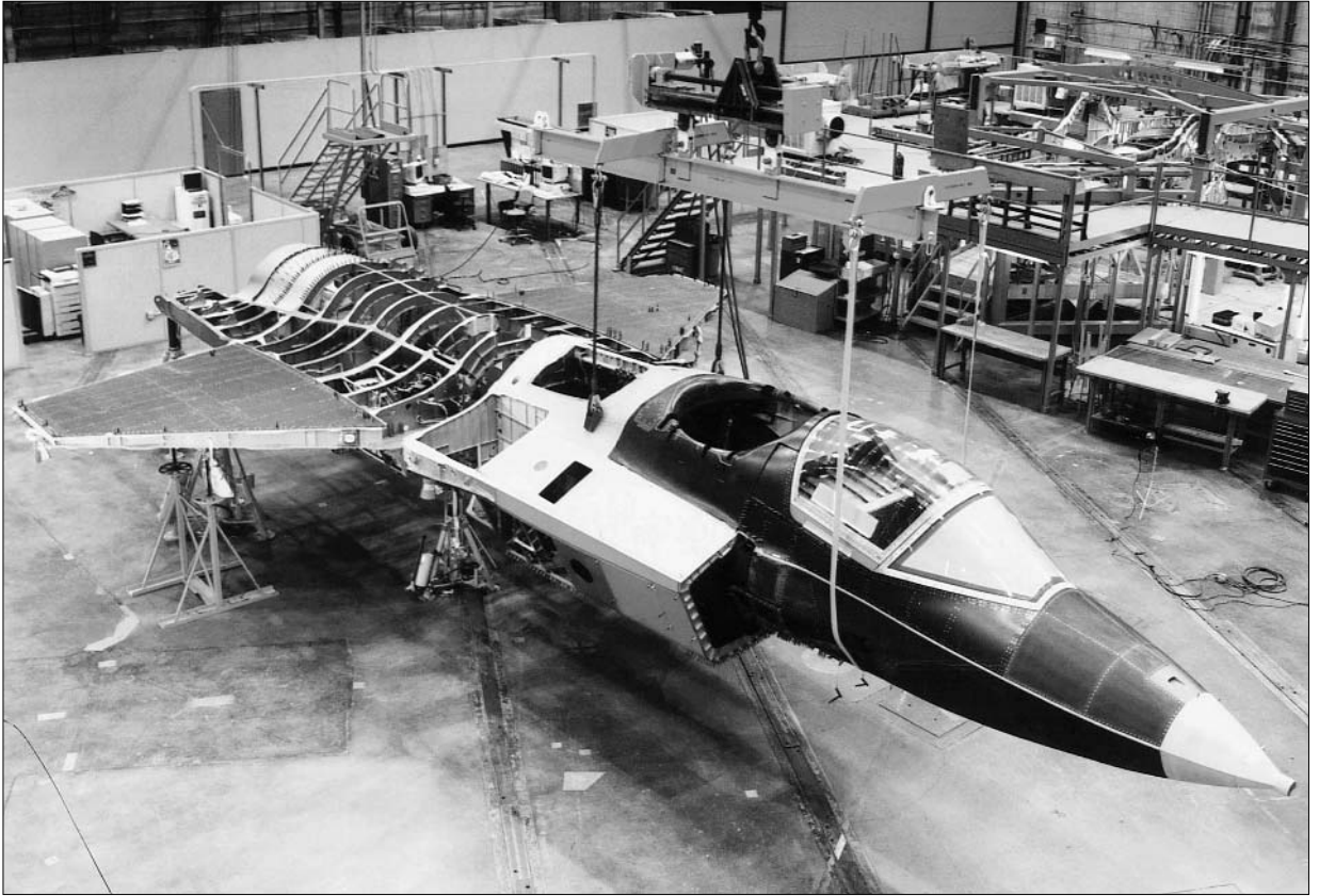
Fig. 10.14(b) X-35 concept demonstrator aircraft after assembly of major structural components (BAE SYSTEMS)
